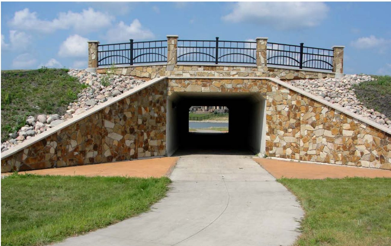
An existing trail underpass in West Fargo
