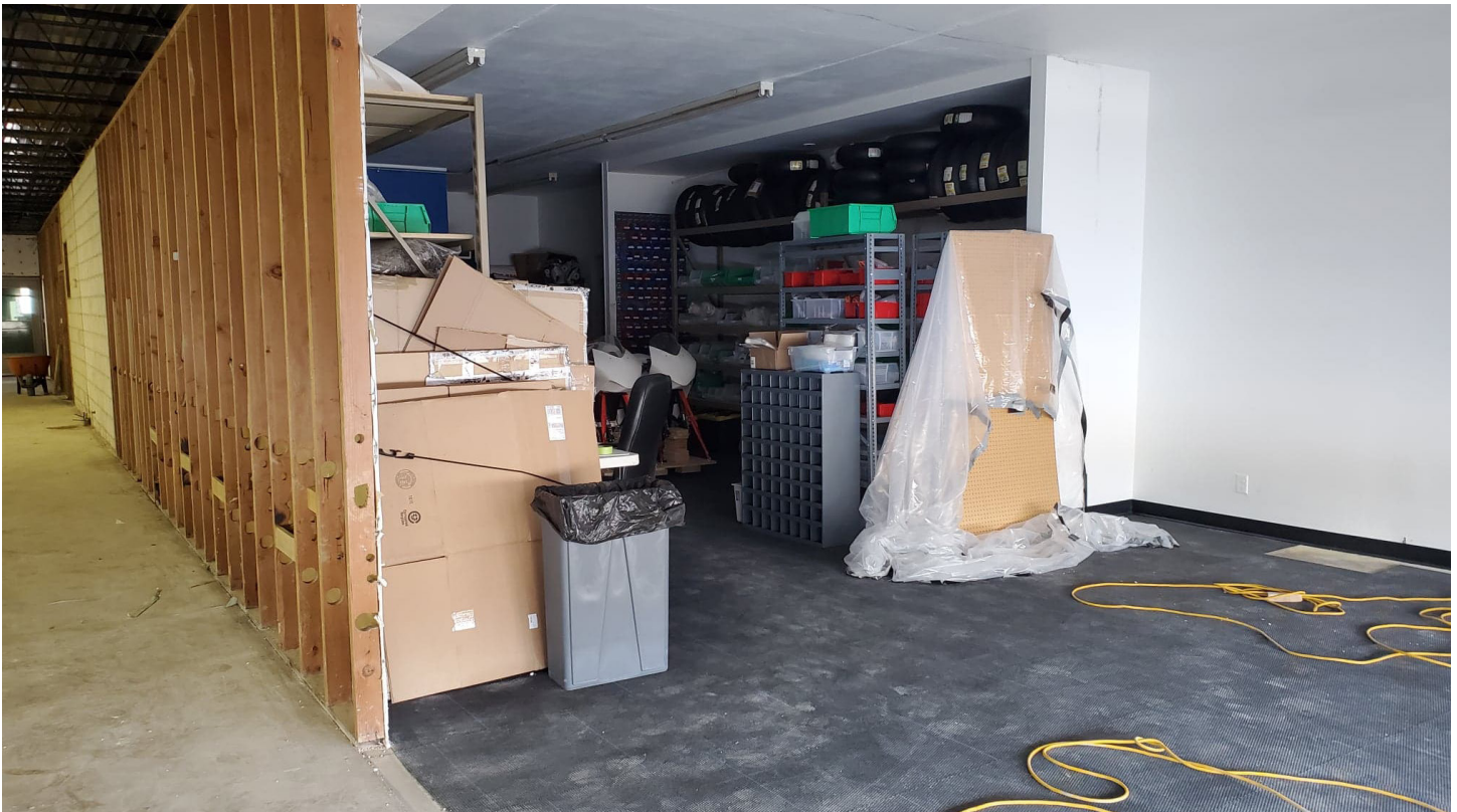
Current Photo looking South West - Standing at Front Door
