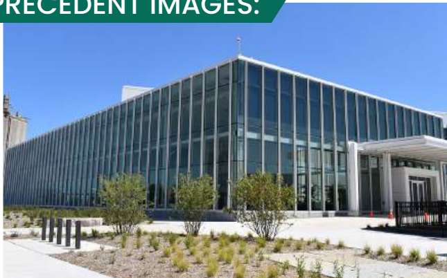
Expanded business park & industrial uses
