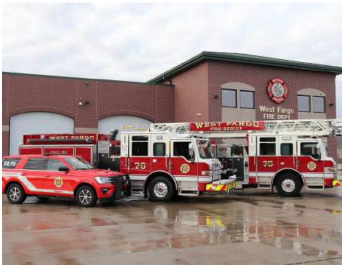
Fire Station/Public Safety Building Could be Integrated With the Landfill Site
