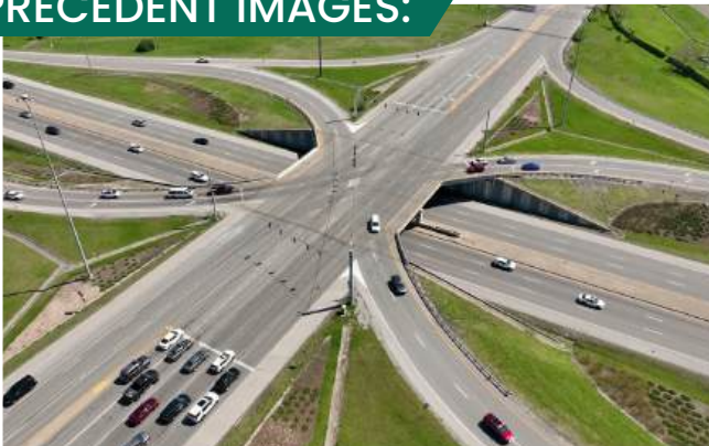
New interchange at 13th Ave W
