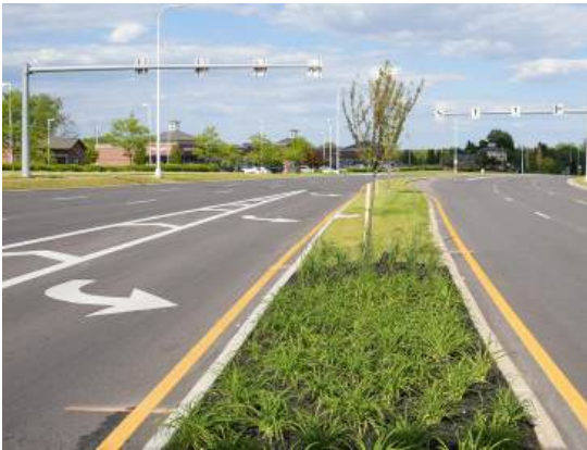
2-3 Lane Collector Roadways
