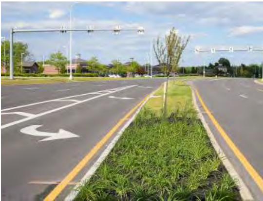
2-3 Lane Collector Roadways
