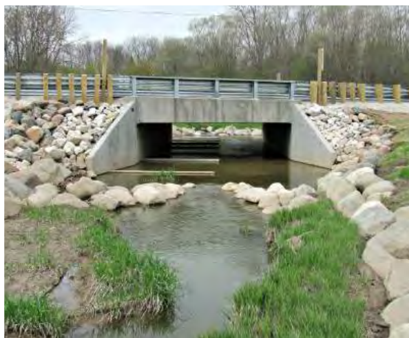
Sheyenne Diversion Crossing Needed
