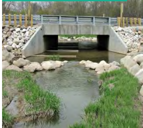
Sheyenne Diversion Crossing Needed
