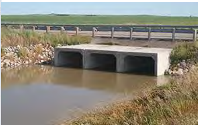
26th Street connection over Sheyenne Diversion
