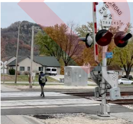
Improved At-Grade Railway Crossings
