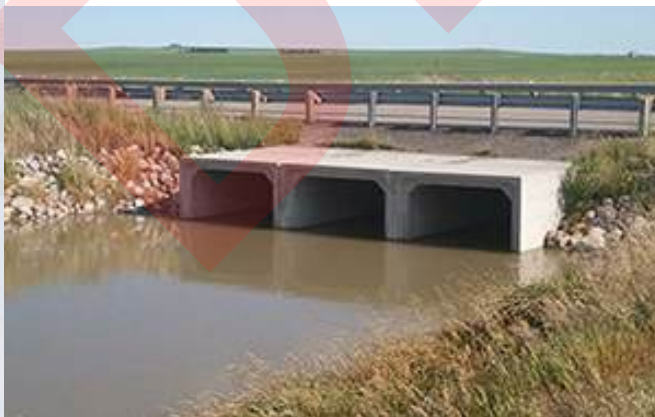
26th Street connection over Sheyenne Diversion
