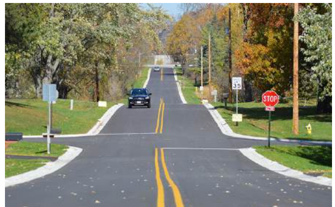
Roadway upgrades to 19th Ave, 38th Street,
