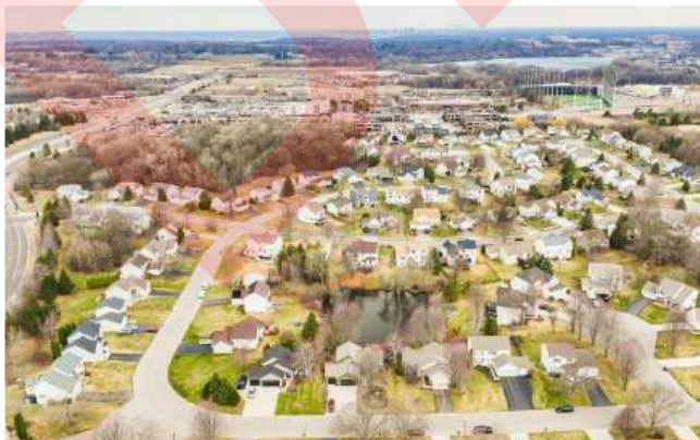
Residential development along the CR 17 corridor
