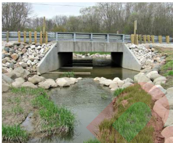
Sheyenne Diversion Crossing Needed
