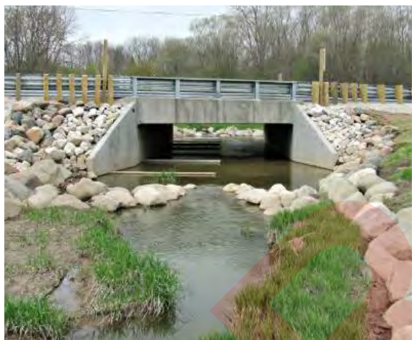
Sheyenne Diversion Crossing Needed
