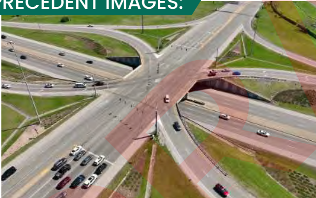
New interchange at 13th Ave W
