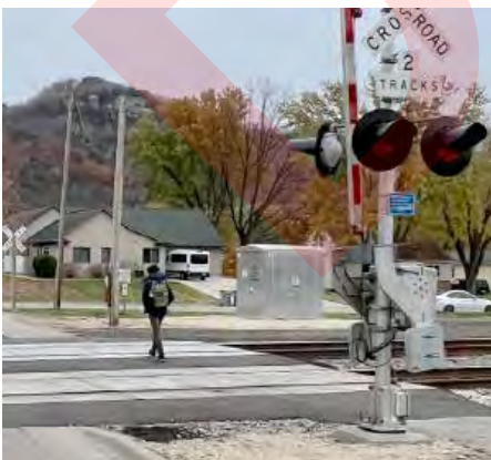
Improved At-Grade Railway Crossings
