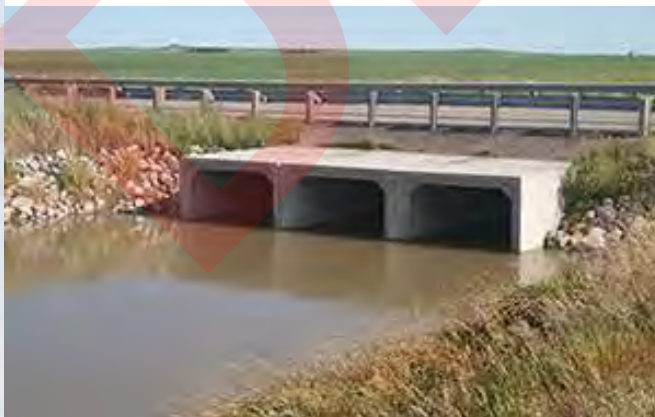
26th Street connection over Sheyenne Diversion
