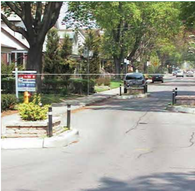
Chicane shifts traffic on a one-way street in Toronto, ON
