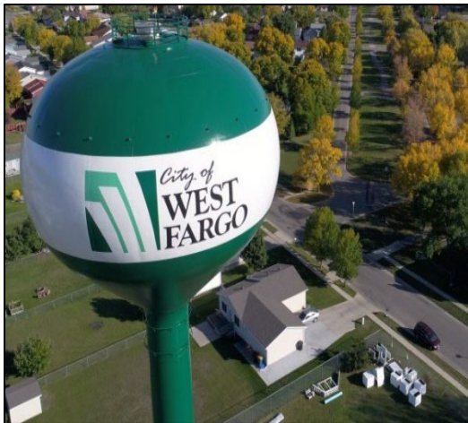
Figure 6 City of West Fargo Water Tower
