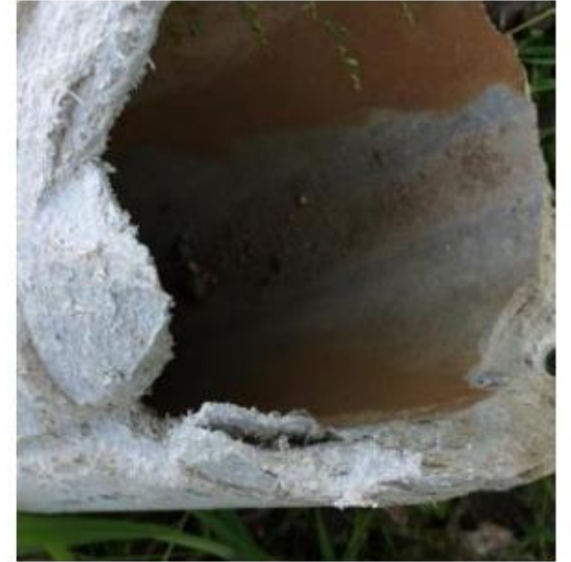
Example Asbestos Cement Pipe
