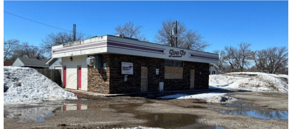
Photo of old Sooper Stop (vacant) at 7th and Sheyenne Streets
