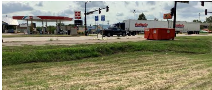
Figure 3: Typical Head Scarp along Main Avenue
